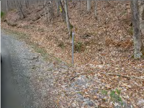
Photo 1: Ditch upstream of cross-culvert inlet on Wilcox Hollow Road is filled in, causing water to follow the road.
