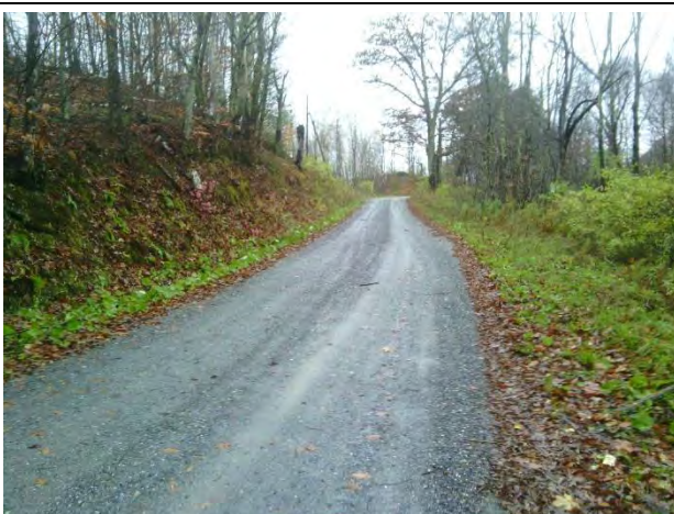
Photo 1: Steep section of upper Wuerslin Road needing stone in ditches and additional cross culverts.
