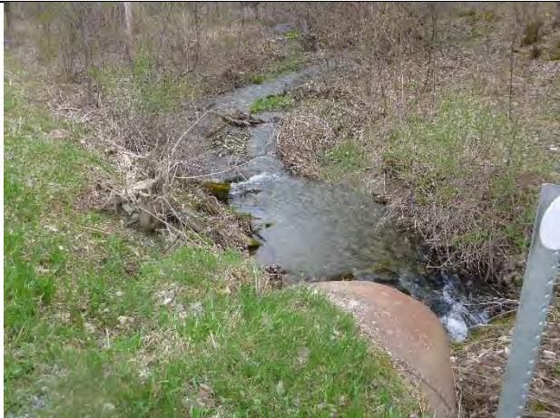
Photo 2: View of downstream channel from roadway. Location of proposed boulder veins to raise tailwater control.
