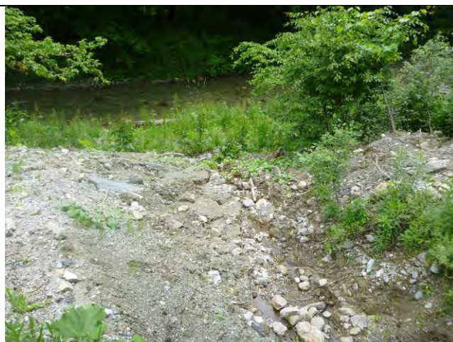
Photo 2: Erosion at a Sandgate Road cross culvert outlet is acting as a source of sediment to the Green River directly downstream.
