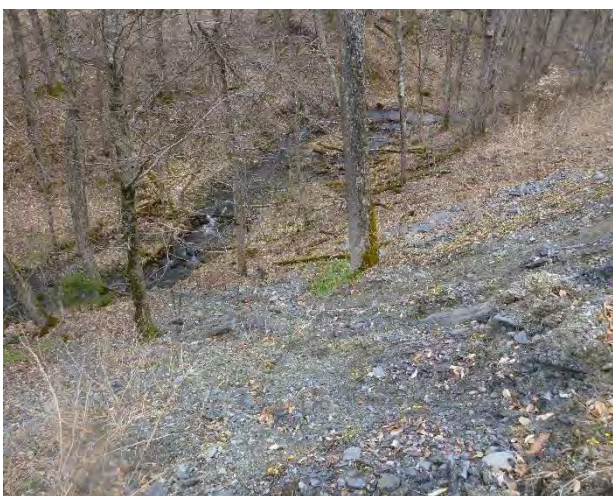
Figure 3: Gully erosion along the steep Rupert Road embankment.
