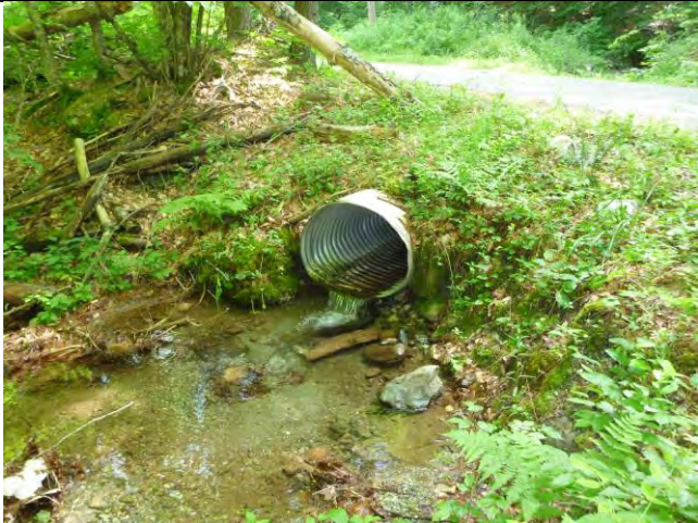
Photo 1: An undersized culvert on Chunks Brook Road.
