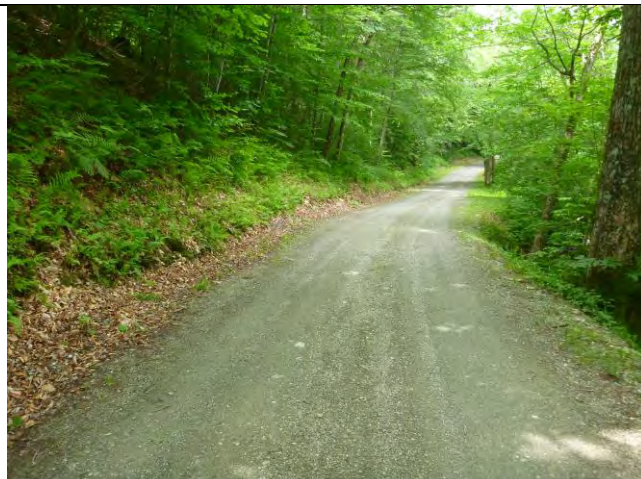
Photo 2: Water currently flowing over the road and eroding the road embankment may be directed into a ditch constructed on the opposite side of the roadway.
