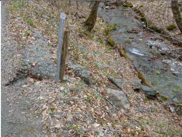
Photo 2: Erosion along the road edge at the cross-culvert outlet adjacent to a second order tributary to the Green River.
