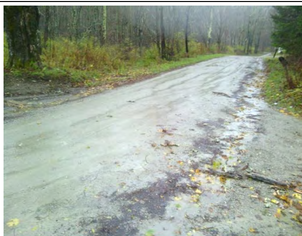
Photo 2: Lower section of Sandgate Road. Runoff is running along the road edge causing rilling and sedimentation downhill.
