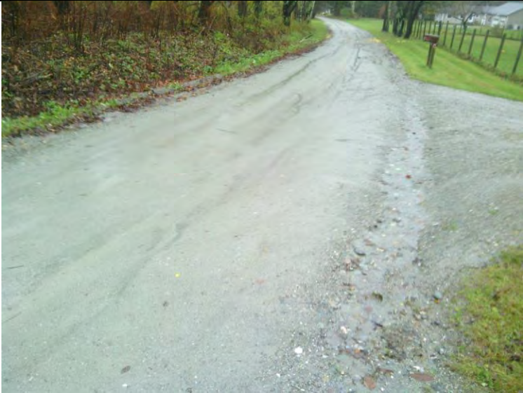
Photo 1: Upper section of Sandgate Road at Woods Gift Lane. Runoff is running along the road edge causing rilling and sedimentation downhill.
