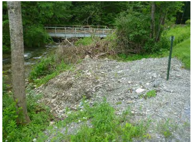
Figure 4: Ditch erosion at a culvert inlet along Woodcock Road (left) was one of the lowest scoring projects (DC-9). Large piles of loose sediment along Sandgate Road (right) following recent culvert and road work were the highest scoring project due partly to its proximity to the stream (DC-14).
