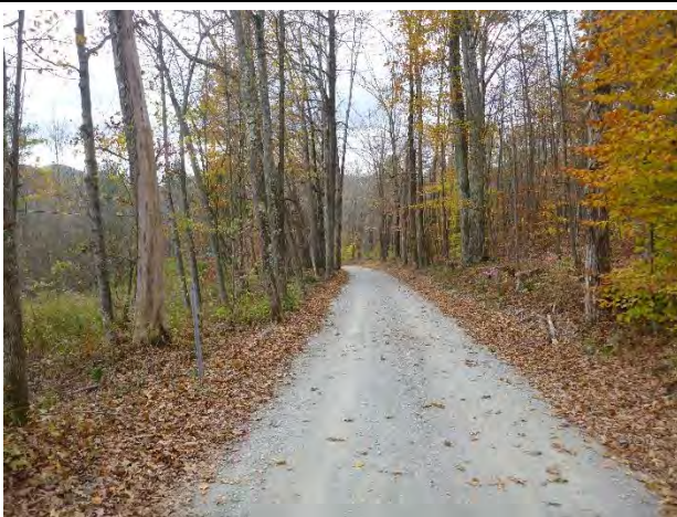
Photo 1: The road has a near continuous tall grader berm (with large trees) along the east side and an undersized and shallow ditch along the west side.
