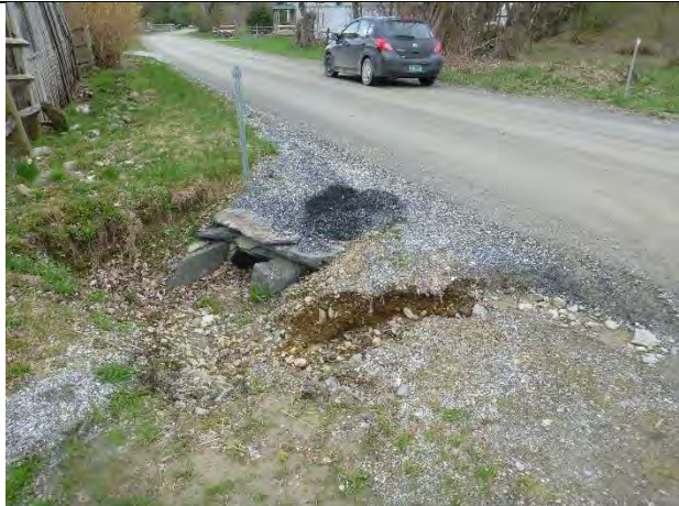
Photo 2: Filled in, poorly defined ditch with erosion where runoff flows along the road over the culvert inlet.
