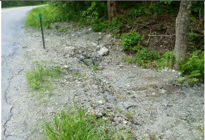
Photo 2: Unstable sediment at a Sandgate Road cross-culvert-inlet.
