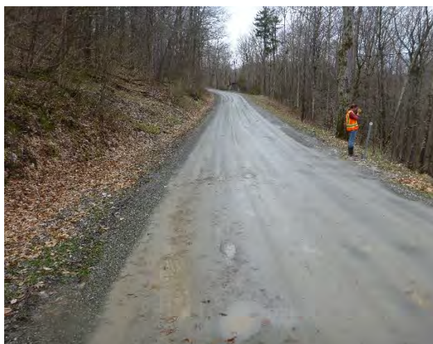
Figure 2: The road crown does not direct water into the existing ditch and cross culvert along a section of Rupert Road.
