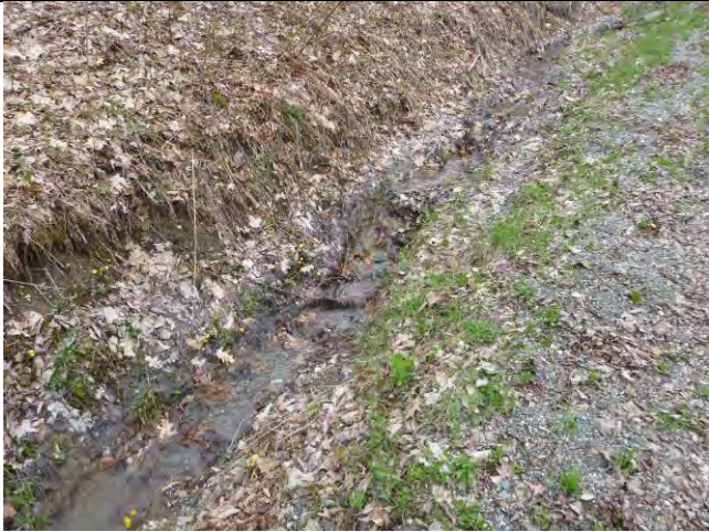
Photo 1: A headcut and erosion in the ditch upstream of a West Road cross culvert.
