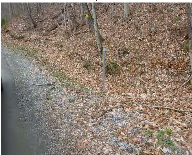
Figure 3: Filling in of the ditch upstream of the culvert may be causing water to spill out of the ditch onto the roadway.
