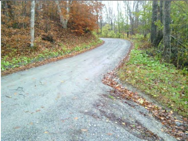
Photo 1: Runoff down a steep portion of Wuerslin Road is causing erosion at the secondary turn to Sandgate Road.
