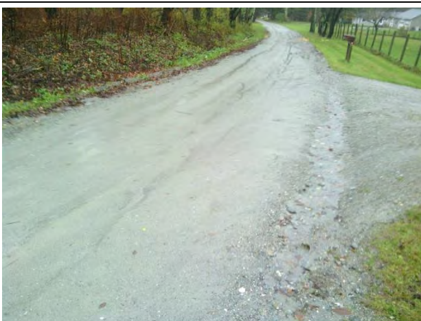
Photo 1: Upper section of Sandgate Road at Woods Gift Lane. Runoff is running along the road edge causing rilling and sedimentation downhill.
