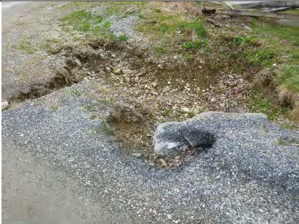
Photo 1: Severe gully erosion along the road edge and at the cross-culvert inlet.
