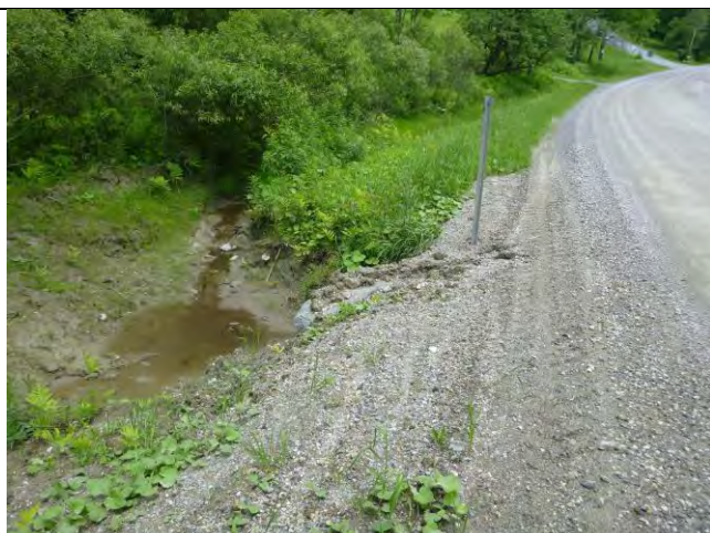
Photo 1: Water flowing over Sandgate Road is causing erosion at a cross culvert inlet, acting as a source of sediment to a roadside wetland.
