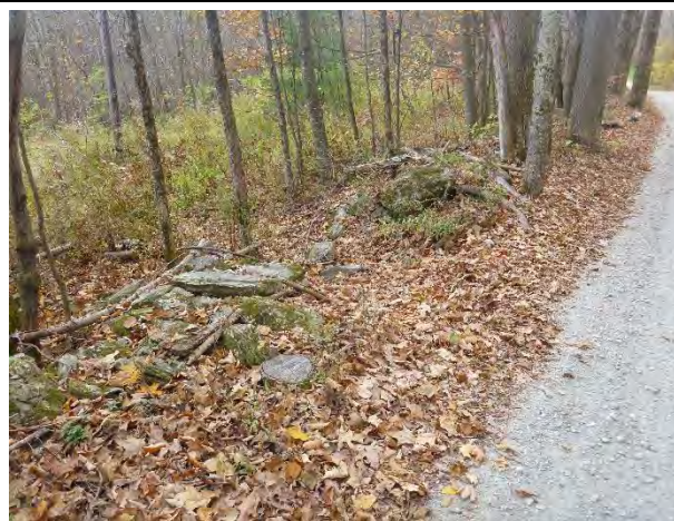
Photo 2: Existing armored turnouts are only partially accessible due to accumulation of road bed material.
