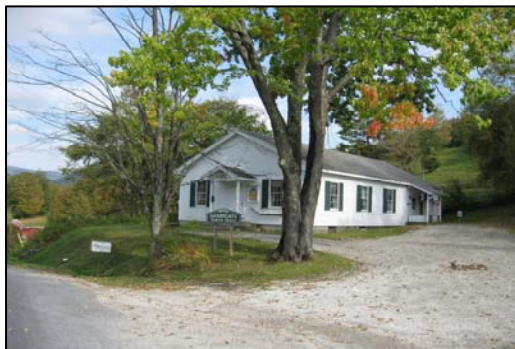
Figure 19: Sandgate Town Office.
