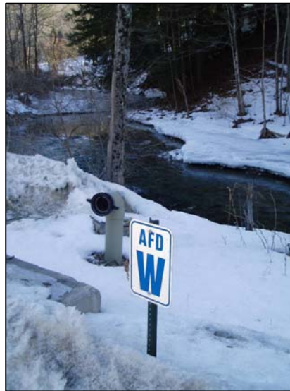
Figure 22: Green River dry hydrant.
