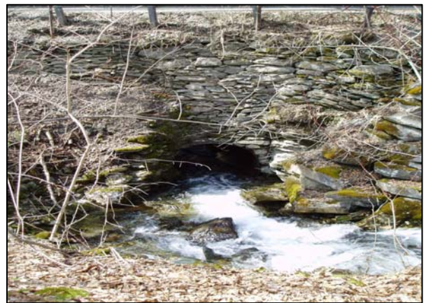
Figure 12: Stone arched bridge on Woodcock Road.
